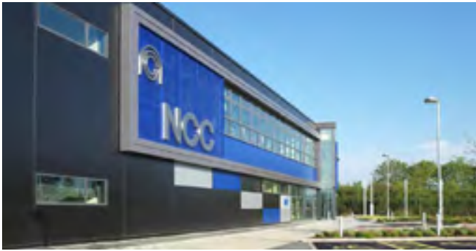
NCC building and workshop facility
